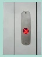
Interlocking system designed for controlling the access to 2 or more doors.
